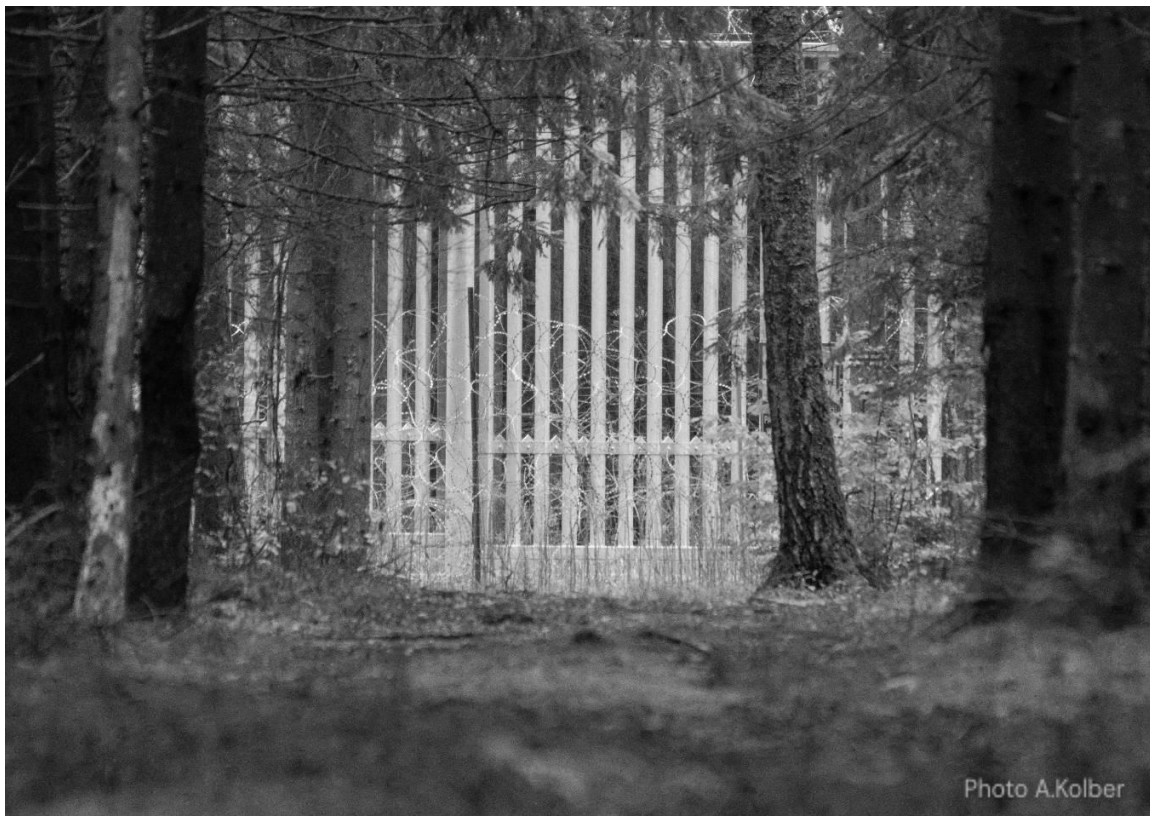
Pic. 1 The image of horizontal elements designed to prevent bending the poles with car jacks.
